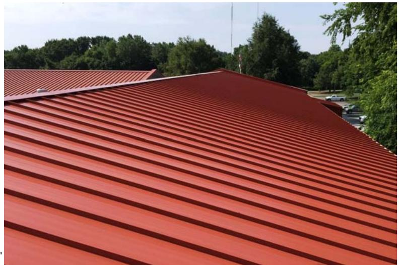
Oil canning: Union Corrugating Company purchases prime commercial grade light gauge metal which is manufactured to all industry accepted tolerances. "Oil canning" is an inherent part of light gauge cold formed panels and is not cause for rejection.
